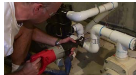
Figure 6. A reciprocating saw often works well to cut PVC pipe during the installation process.
