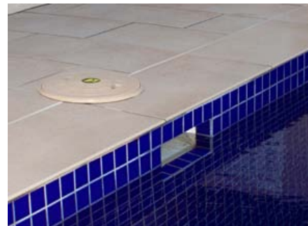
Figure 9. The skimmer is the port that draws water from the pool and into the filtration system.
